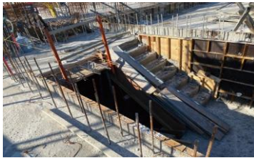
[Leading edge of slab 슬래브 단부]
