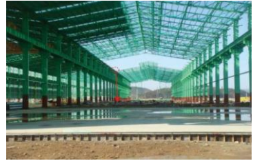
[ Newly constructed factory roof (panel) ]
