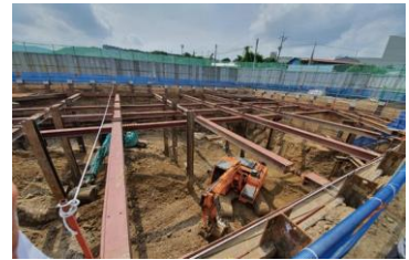
[earth retaining structure (spread beam)
