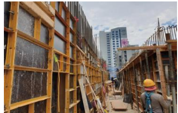
[Formwork (Euro form) 거푸집(유로폼)]
