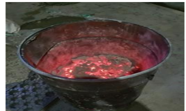
[Place for brown coal curing of concrete 갈탄콘크리트양생장소]
