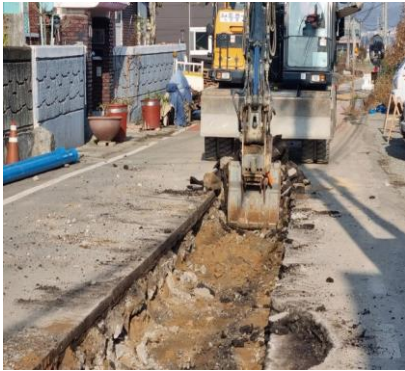
Excavation work 굴착작업
