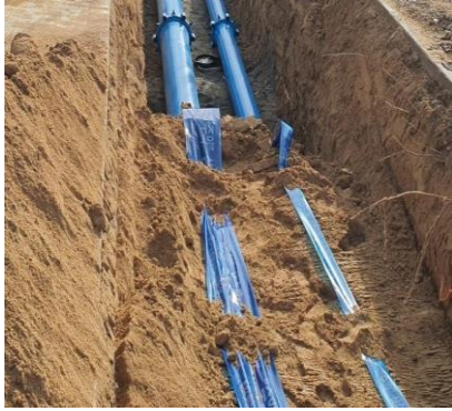
Backfill after burial of pipeline 관로매설 후 퇴매우기
