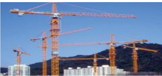
[T-type tower crane T-형 타워크레인]
