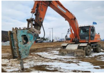
[Breaker-installed excavator 브레이커장착굴착기]
