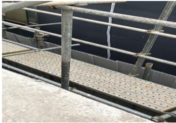
[Work platform 작업발판]
