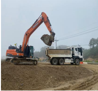
Transporting excavated earth/sand 토사운반
