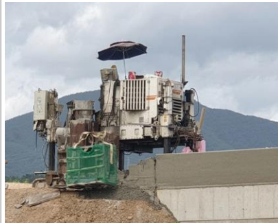
Installation of protective wall 방호벽 설치
