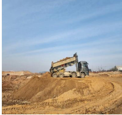
Shipping-out of earth and sand 토사반출
