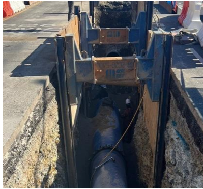
Installation of sheathing timbering 흙막이설치
