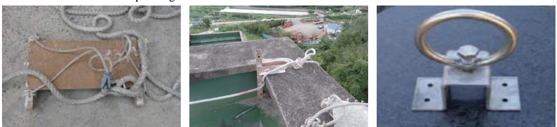
[Hanging scaffolding work platform 달비계작업대] [Rope knots 로프매듭] [Hooks for ropes to hang on 로프걸이용고리]
