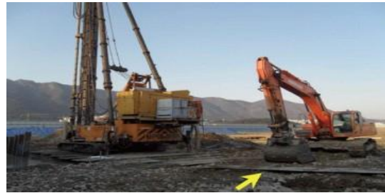
[Pile driver (soil-retaining file driving) 항타기(흠막이파일박기)]
